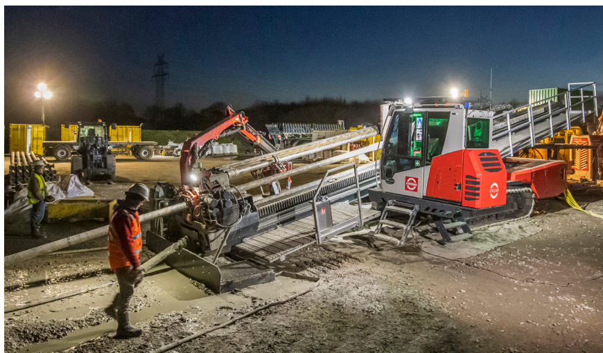
Figure 1. HDD80-E rig is field-tested within e.g. projects of trenchless laying of electric power lines.
