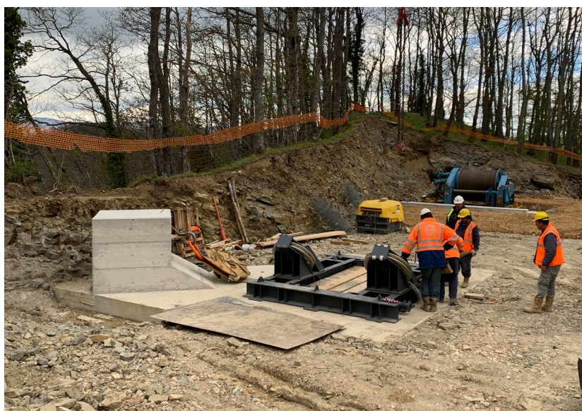
Figure 4. Preparing the pipe installation from the ridge: anchor block (left) and steel frame (middle) with pulleys.
