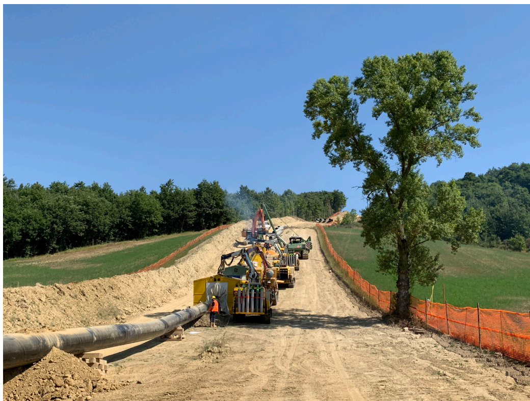
Figure 2. Automatic welding.
