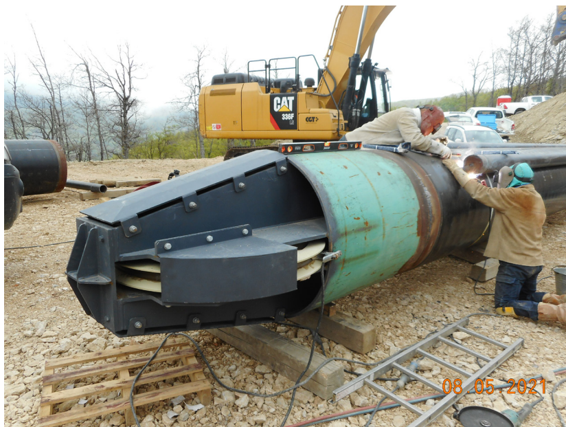
Figure 3. Launching head with welded first piece of pipe.
