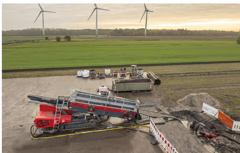
MAX STREICHER: HDD45-E on site.
