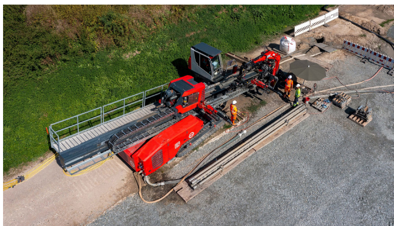
MAX STREICHER: HDD80-E on site.
