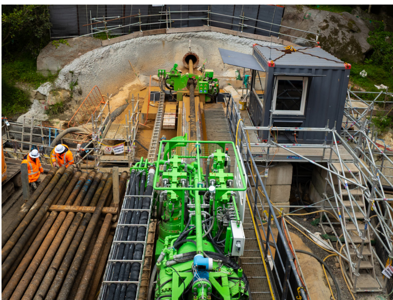
Herrenknecht: HDD Rig HK250C, on-grade pressure sewer pipeline for Refresh Vacluse and Diamond Bay project for UEA Pty Ltd, Australia.
