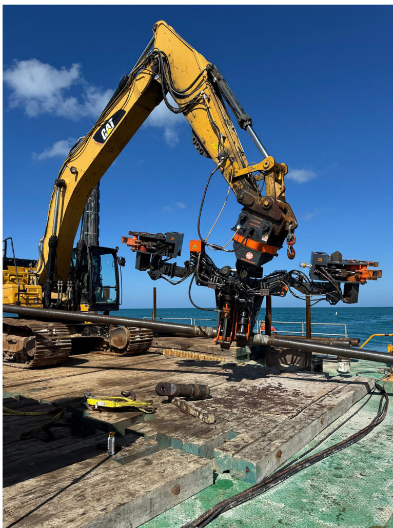
LaValley Industries: Mechanised system maintaining positive grip, alignment, and controlled torque to support predictable and repeatable handling of pipe and tooling during HDD exit-side operations.
